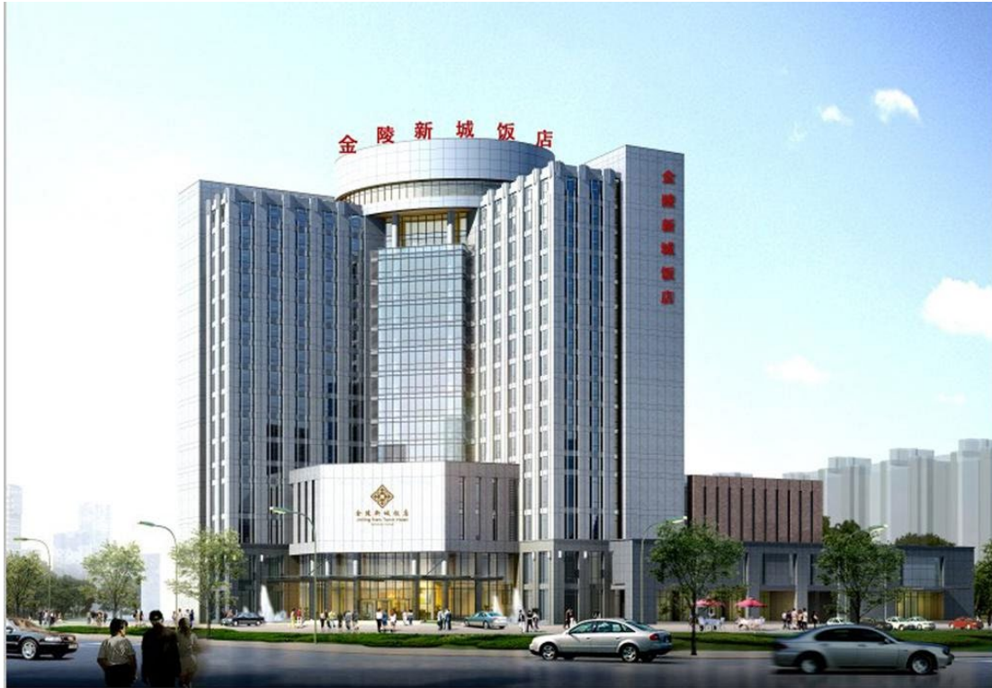
Fig. 4 Jinling New City Hotel Nanjing
